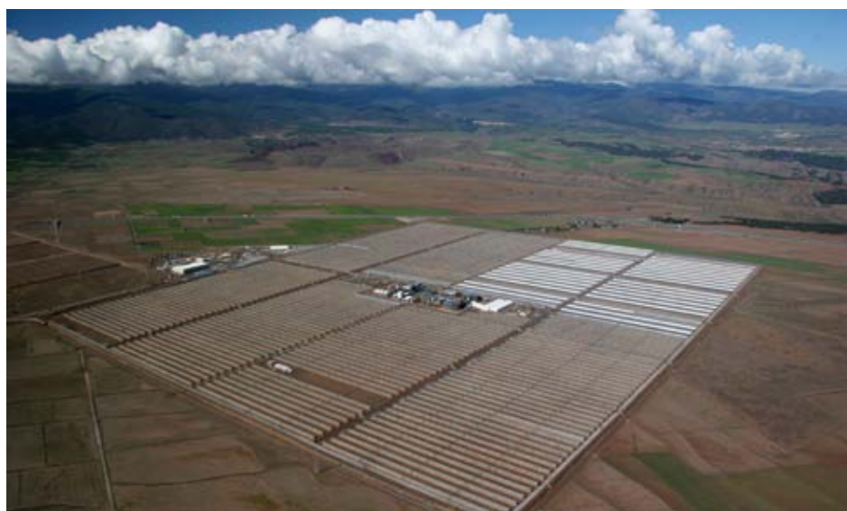
Andasol 3: HORA has succeeded in entering the solar thermal power plants sector!
