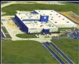
PAGELAND, SC Bronze Foundry and Manufacturing Plant
