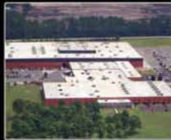
CONWAY, SC Steel Foundry and Manufacturing Plant
