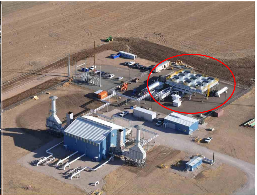
Above top left: modular assembly produced on the shop floor; Left: ORC skid being loaded onto a truck for transportation to a project site; Above: a 4MW waste heat installation on an existing dual-turbine gas compression site (the ORC system and its heat rejection is circled in red)
