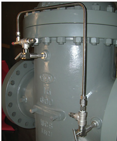
SCV installed Thermal Relief system on 16" Class 600 Thru Conduit Gate Valve
