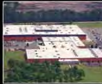
CONWAY, SC Steel Foundry and Manufacturing Plant
