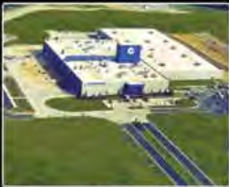
PAGELAND, SC Bronze Foundry and Manufacturing Plant
