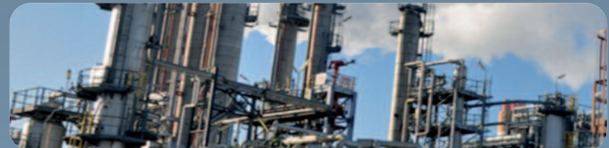
Improving plant safety, reliability and efficiency
